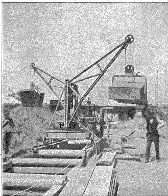
FIG. 287.—Engine-driven crane, by the Motorenfabrik "Oberursel."
