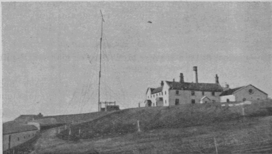
Fig. 37. — Station de South-Foreland.
