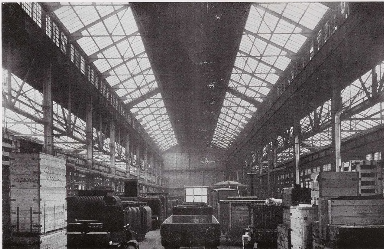
Metropolitan-Vickers Electrical Co. Ltd., Trafford Park, Manchester.
