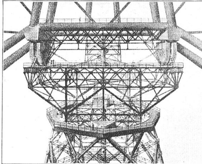
FIG. 6. — AU SOMMET DE LA TOUR QUI SUPPORTE LES ROUES ÉOLIENNES
