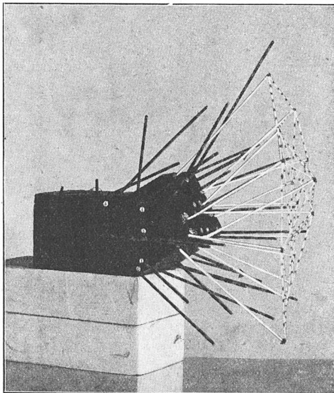
FIG. 6. — LES DERNIERS SONDAGES AVANT L'EXPLOSION FINALE LORS DU PERCEMENT DU LAC D'ARAING
